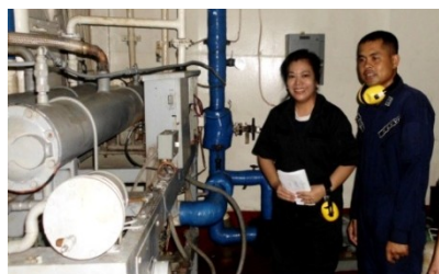
Main Auxiliary Starboard
